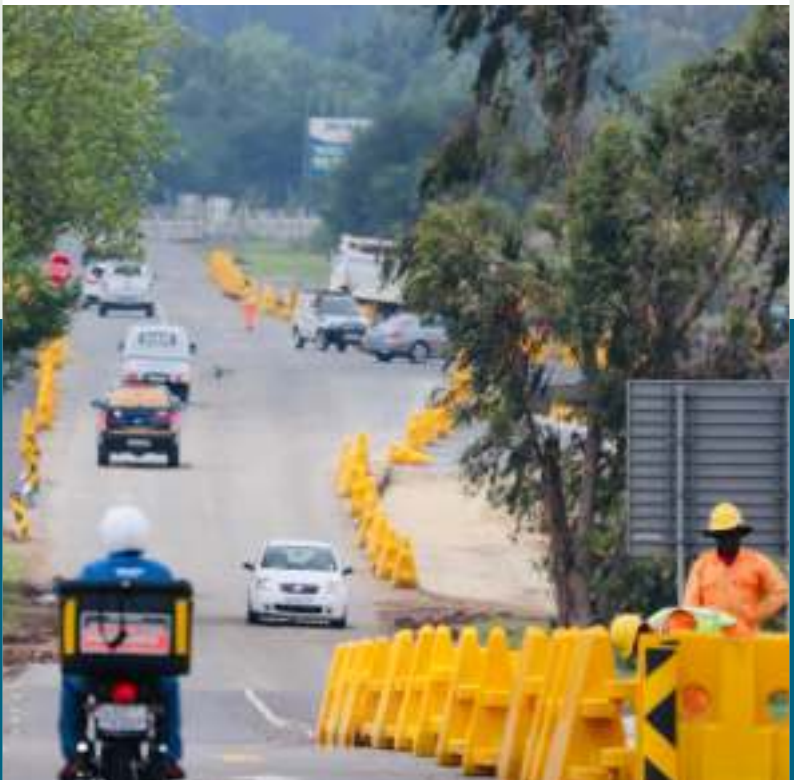
Upgrading of roads near North West University Vaal Campus
